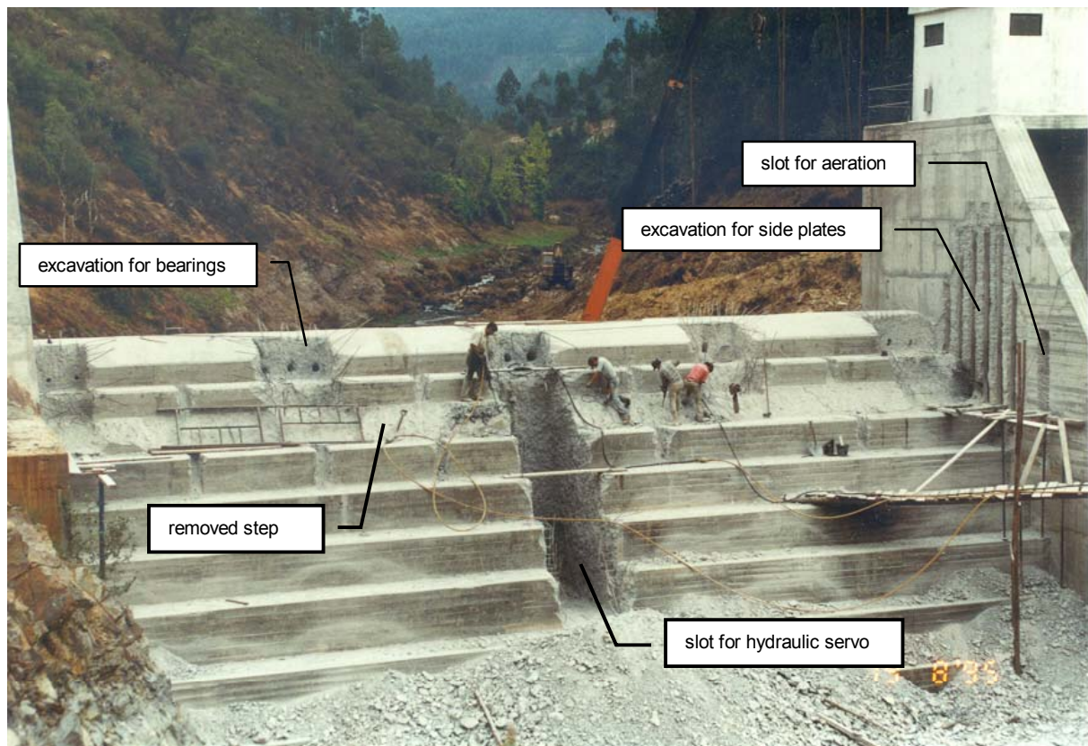
Fig. 11: Work on Spillway in Progress
