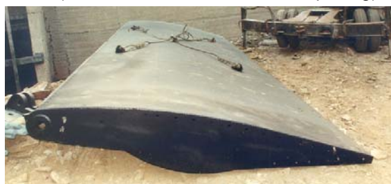
Fig. 9: Section with Flap Gate (with Side Plate and Aeration Opening)
