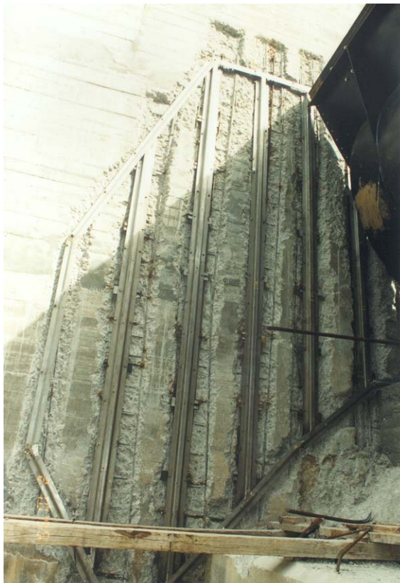
Hat-Profiles, mounted to the wall
