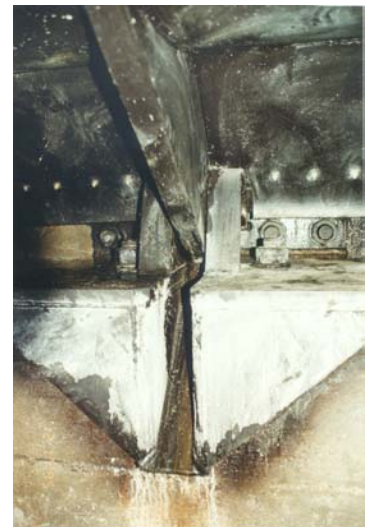
Fig. 6: Bearing Box with Slot
