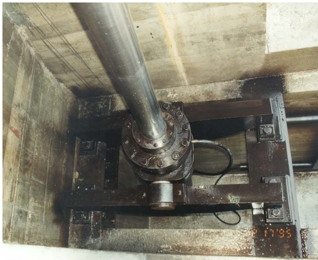
Fig. 5: Bracket for Hydraulic Servo
